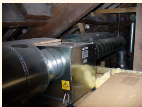
Settle Meeting House has two air exchange units which recycle hot air at ceiling level, reducing energy needs. Photo: Michael Elstub
