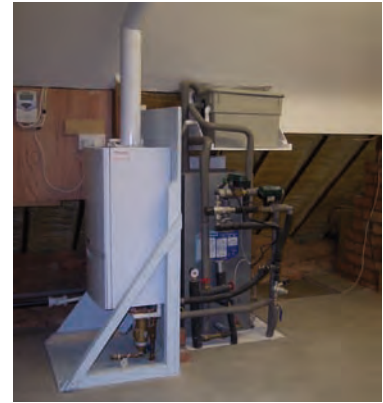
A condensing combi boiler located near a solar heated 'heat store'. Photo: Tom Greeves
